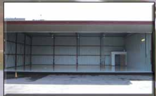
RESTROOM IN EACH UNIT
